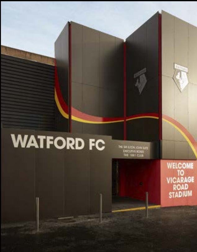
Watford Football Stadium Hertfordshire, United Kingdom
